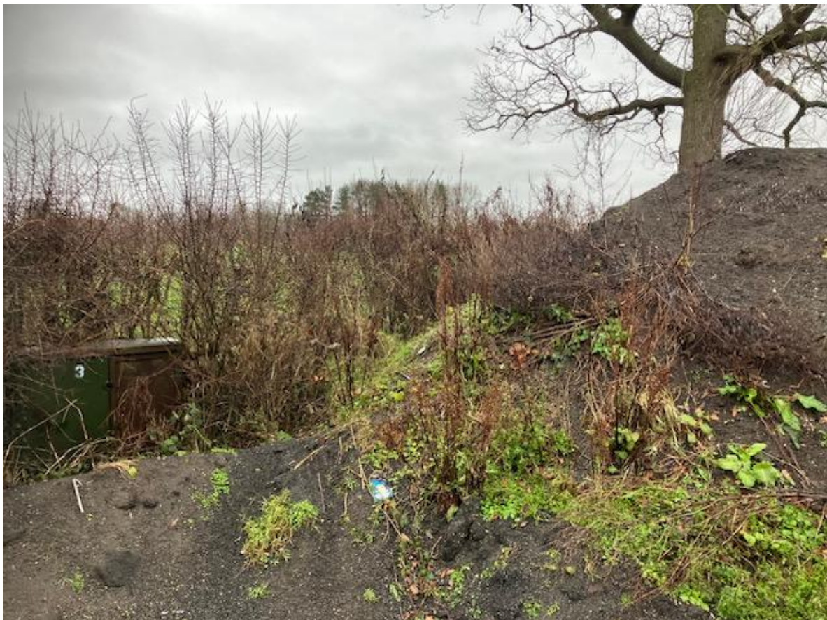
Green fibre optic cabinet on the left of the picture.
