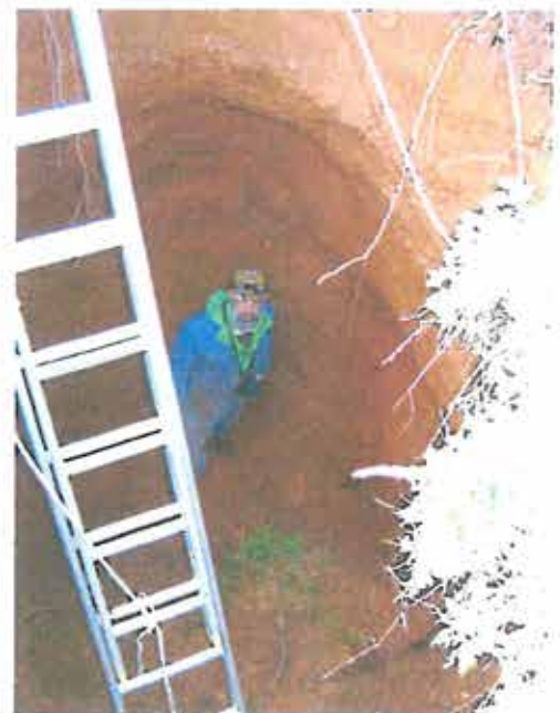
Figure 17 Jim down the hole
