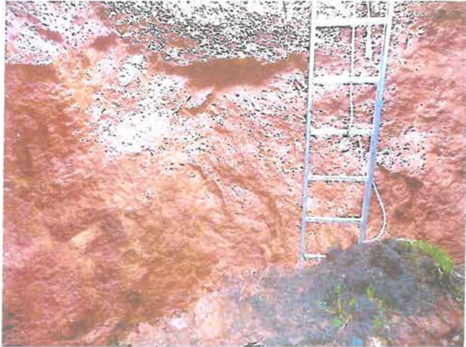
Figure 18 Side of the hole looking up from the bottom with ladder on fallen in surface material
