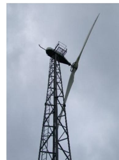
At Yew Tree Farm at Drointon a mid size wind generator is teamed with a solar farm and, because the peak operating times for wind and solar systems occur at different times of the day and year, the system is more likely to produce power when you need it.
